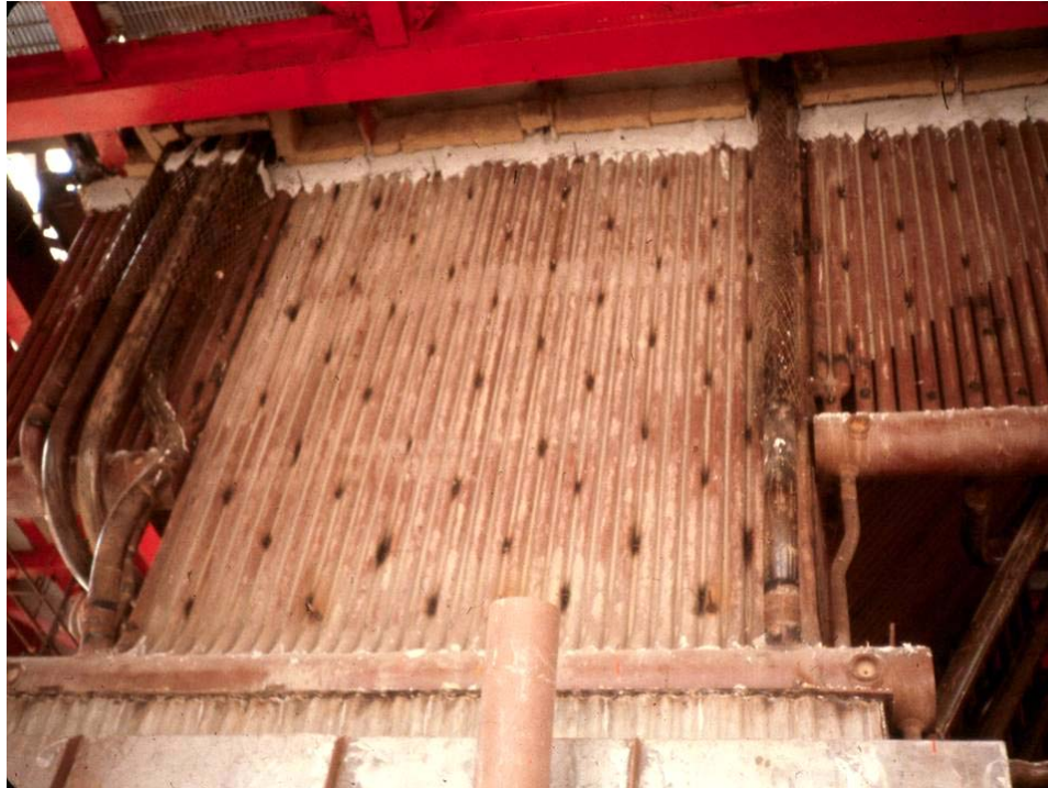
Figure 3-1. Waterwall Furnace Section 9
